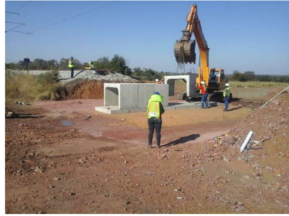
Figure 17 Construction of culverts during Transnet's 2018 mid-year shut down maintenance period
