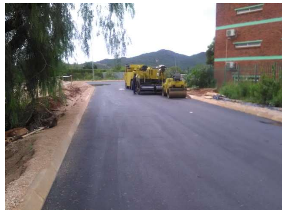
Figure 10 Asphalt Seal at Ga-Rankuwa
