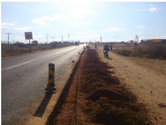
Excavation of the edge beam
