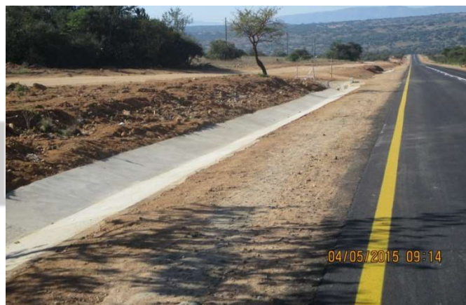
Photo 4 Complete Road and Concrete V drain
