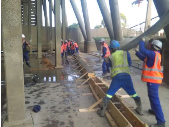
Figure 7 Casting of Concrete at Cooling Tower 1
