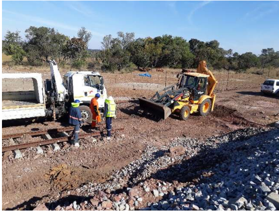
Figure 16 Delivery of culverts
