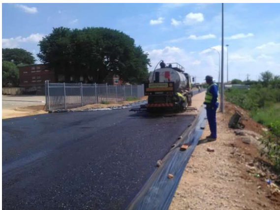
Figure 9 Prime Coating at Ga-Rankuwa
