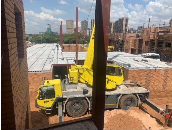
Photo 1 Construction of Apartments in Marabastad, January 2020.
