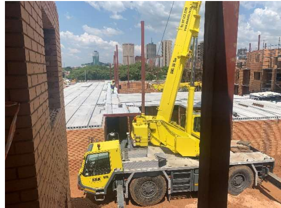
Figure 21 Loading of precast Slab
